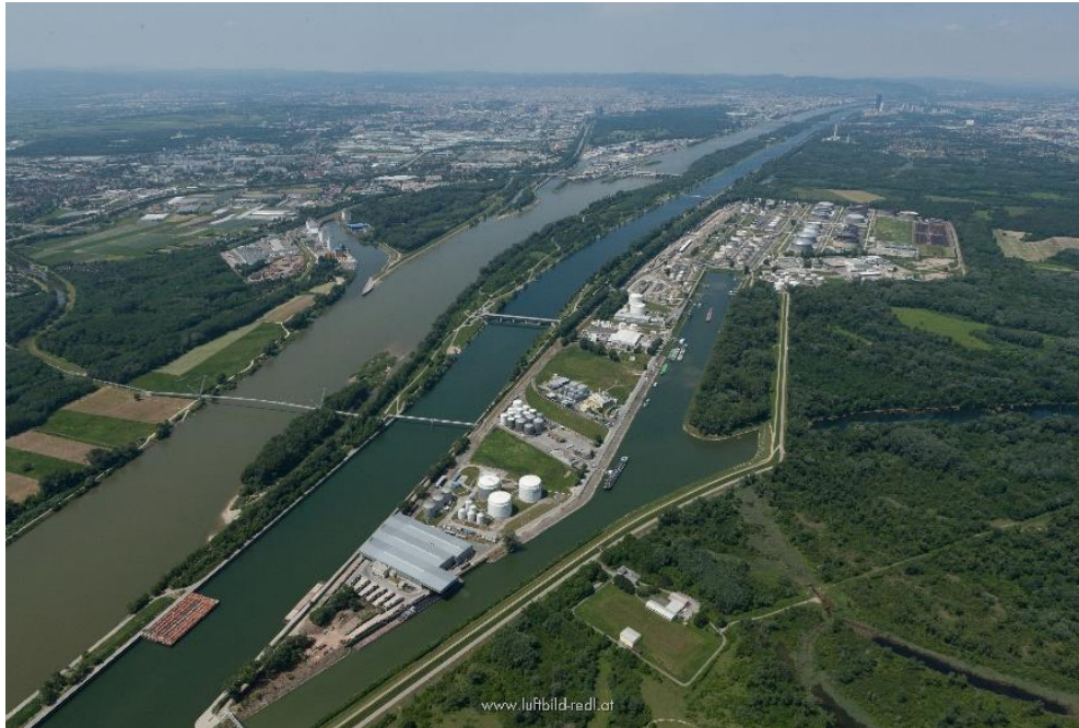
Figure 8.: Port of Vienna – location Lobau
