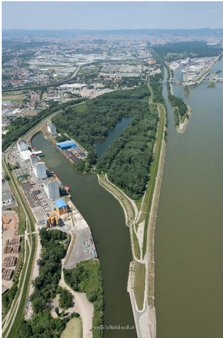
Figure 7: Port of Vienna – location Albern (Source: www.hafen-wien.com )
