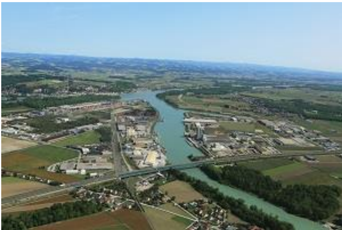
Figure 2. View of the Ennshafen Port (Source: EHOÖ)
