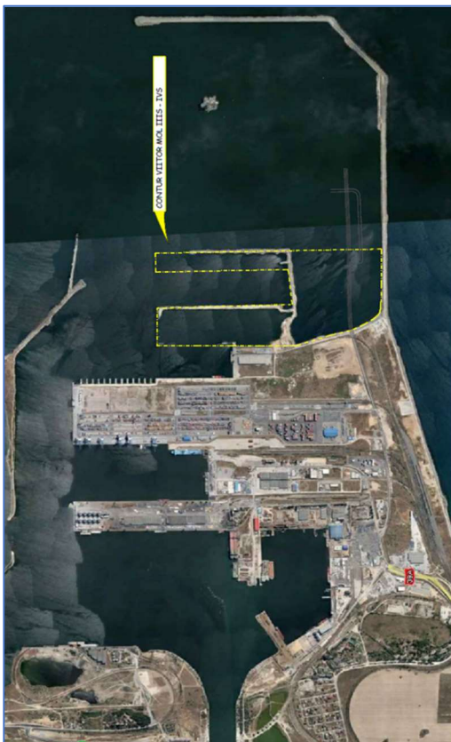
Figure 11.8: Dredging in the Port of Constantza, the Midia area and the Port of Mangalia (including the widening of the access mouth)
