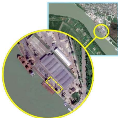
Figure 14.13: Construction of complex for processing mineral fertilizers on 8th berth and the rear zone on the territory of the production and transshipment complex No 1 SE "Izmail State Merchant Sea Port".
