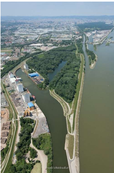
Figure 6.11: Port of Vienna – location Albern (Source: www.hafen-wien.com )
