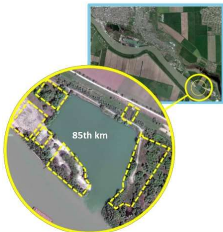
Figure 14.12: Construction of a complex of facilities for transshipment and storage of general and bulk cargo on the section of 85 km of the Danube.
