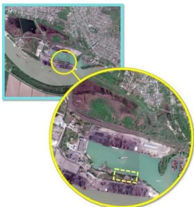
Figure 14.15: Construction of a transshipment complex for bulk cargo in the southern part of the bucket 90 km (two berths, No 27-28)
