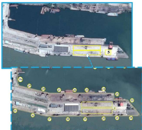
Figure 14.5: Construction of a complex of temporary warehouses
