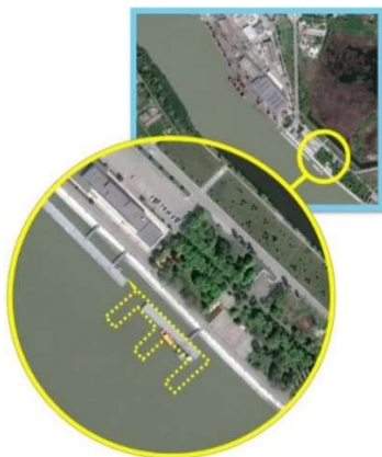
Figure 14.14: Construction of modern marina for small vessels
