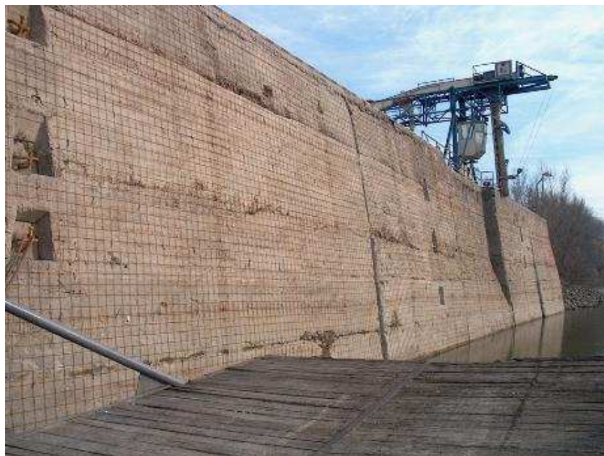
Figure 32: Vertical quay with loading facility for grains
