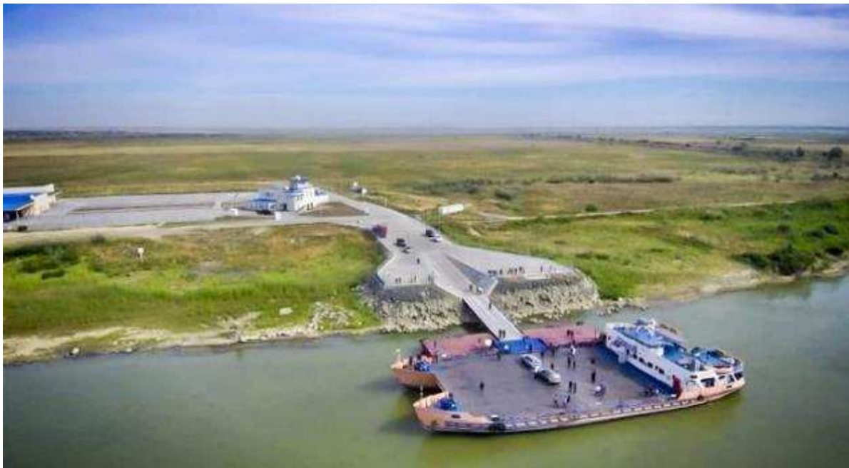
Figure 95: Ferry crossing "Orlovka-Isakcha"
